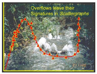
monitoring and notification of potential overflows. Baltimore is embarking on an overflow monitoring effort that will rely heavily on expert interpretation of scattergraphs to detect and quantify SSOs.
