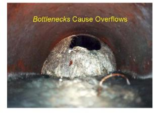
"bottlenecks". "Bottleneck" is a convenient term for a localized decrease in the slope of the hydraulic grade line that attains a slope less than required for proper operation. Sources of bottlenecks that cause overflows include:
