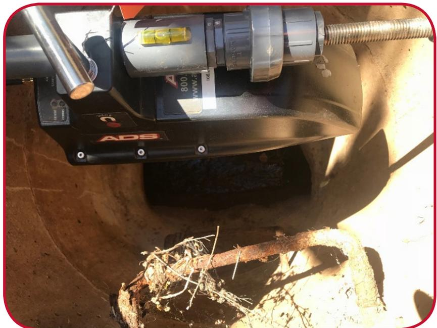
ECHO installation with tension bar makes installation fast and easy.
