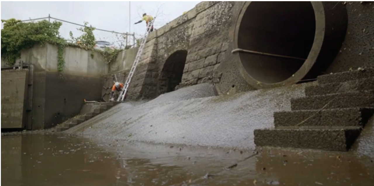
ADS personnel installing remote monitoring systems
