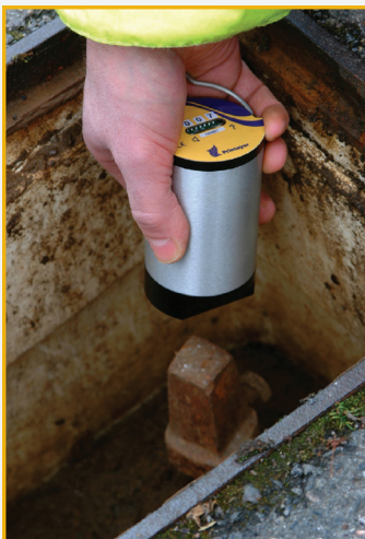
ADS Enigma Pod - Installation on Water Meter.
