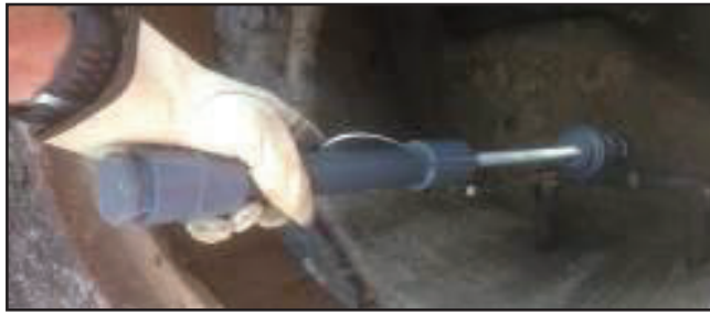
Passing un-tethered end through large loop
