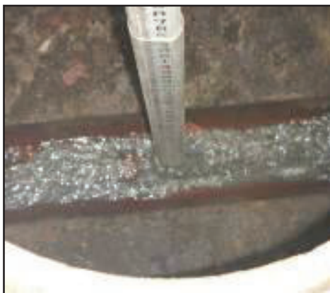
Extending Grade Pole to absolute bottom surface of invert
