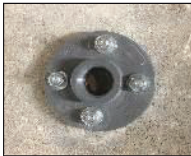
Securing bracket to the manhole wall
