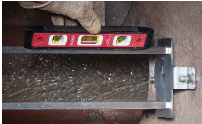
Confirm Level Front to Back
