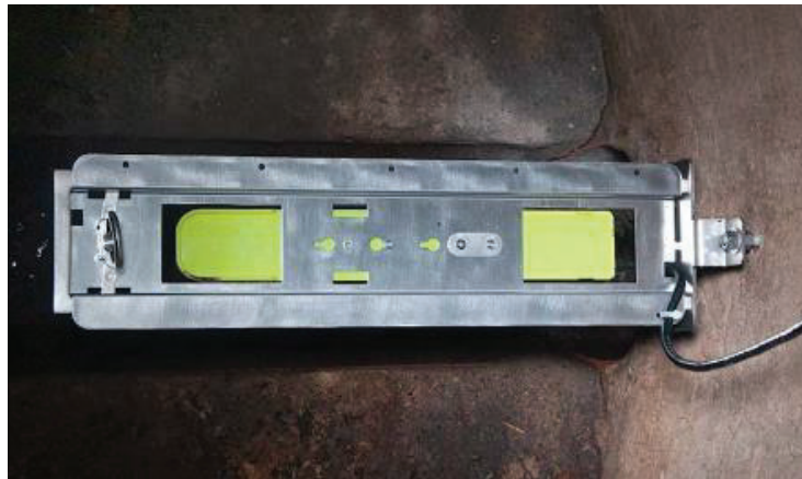
Installed Sensor Bracket on Wall Mount Bracket
