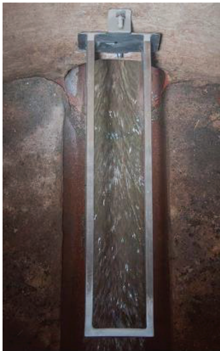
Installed ParaDepth/ParaFlow Wall Mount Bracket
