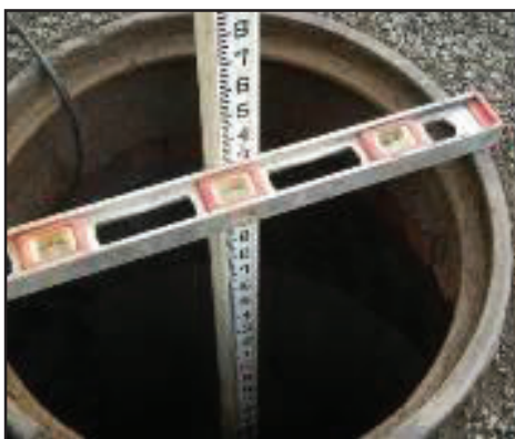
Placing Carpenter's level across open manhole frame
