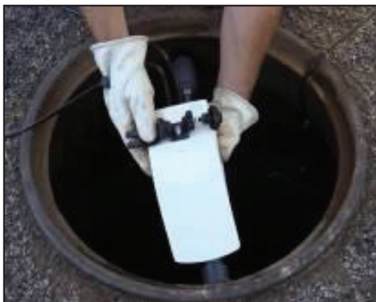
Unscrewing and opening shroud bracket
