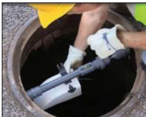
Positioning and tightening sensor bracket to Mounting Bar
