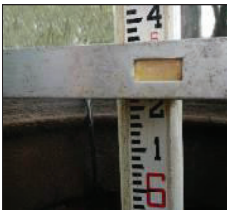
Recording measurement for manhole depth
