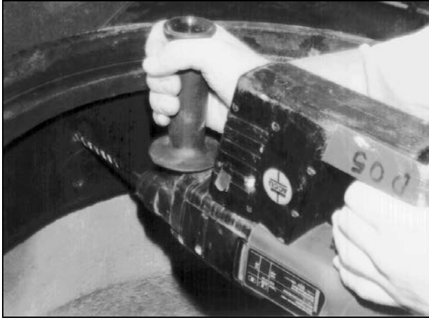
Drilling the hole in the manhole rim
