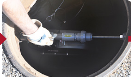
3.2 Lower and Place ECHO on Mounting Bar
