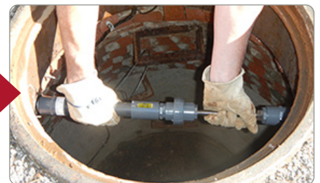
2.6 Expand, Level, and Confirm Secure Positioning of Bar
