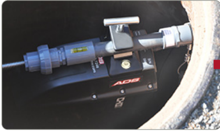
3.4 ECHO Fully Installed
