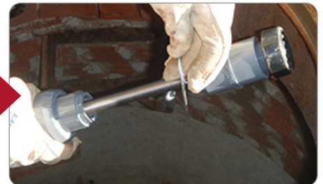
2.3 Pass Untethered End Through Large Loop
