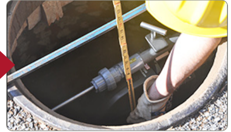
3.6 Measure Distance from the Rim of the Manhole to the Face of the Sensor, Record the Physical Offset Value
