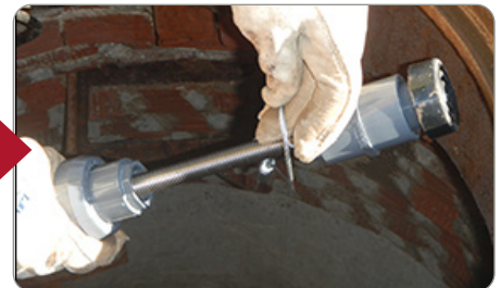
2.3 Pass Untethered End Through Large Loop
