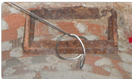
2.4 Pull Tether Tight, Cinching to the Top Rung
