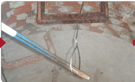
2.2 Use J-Hook to Pull Tether up from Top Rung
