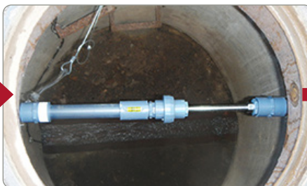
2.5 Ensure Bar Installation Gives Clear Line of Sight to the Invert
