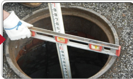
1.2 ...to the Manhole Rim, and Record the Manhole Depth Value
