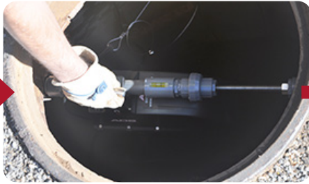
3.2 Lower and Place ECHO on Mounting Bar
