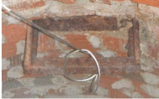
Cinching Tether to the Top Rung
