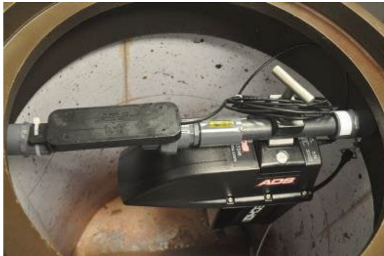
In-manhole antenna installed to mounting bar
