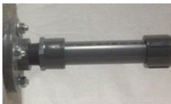
Screwing Wall Mount Bar into Installed Bracket
