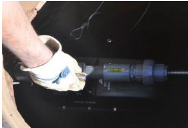
Placing Monitor on Mounting Bar
