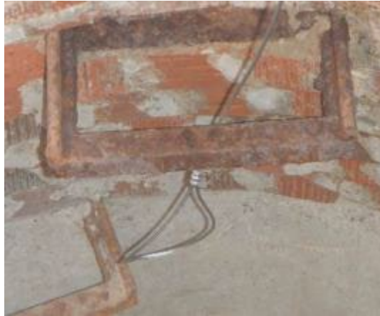
Passing Mounting Bar Tether Behind Top Rung
