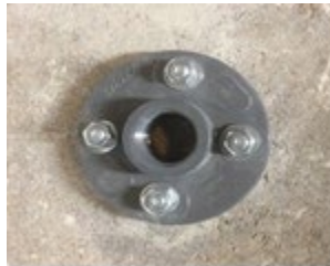
Securing Bracket to the Manhole Wall
