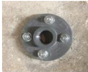
Securing Bracket to the Manhole Wall
