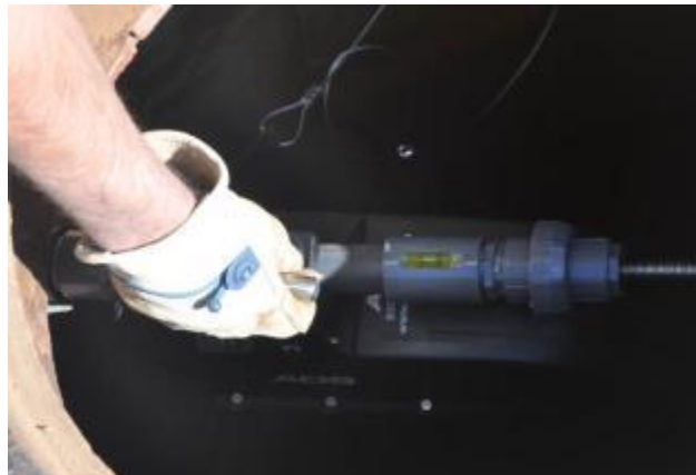
Placing Monitor on Mounting Bar
