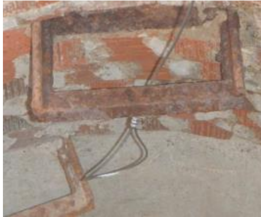
Passing Mounting Bar Tether Behind Top Rung
