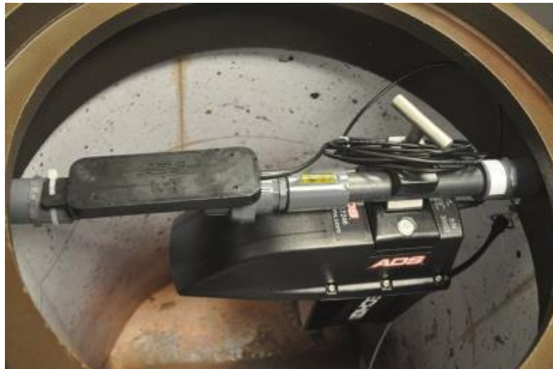
In-manhole antenna installed to mounting bar
