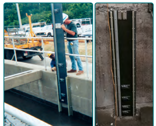
7658 Transducers Mounted on Sliding Plates
