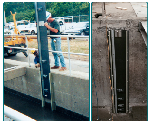
7658 Transducers Mounted on Sliding Plates
