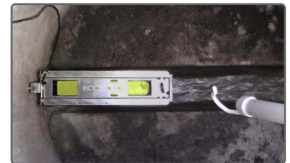
PARAFLOW installed in a manhole with Topside Retrieval System
