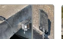
**4.5** Install antenna flat with logo up with unobstructed view of sky or tower. Place antenna a minimum of 1 ft from the unit.
