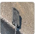
2.8 Install antenna flat with logo up with unobstructed view of sky or tower. Place antenna a minimum of 1 ft from the unit.
