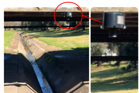
FS-UL monitoring storm channel level
