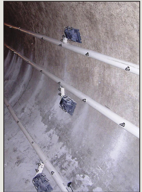
Internal mount pipe installation with cable conduit
