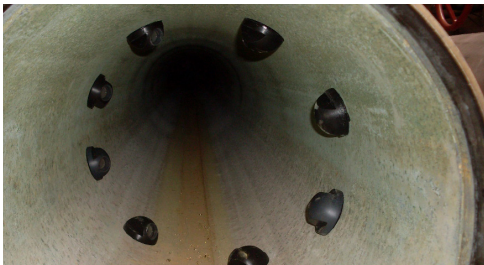
7625 Transducers Installation - Internal View
