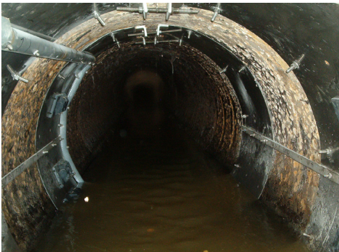
7658 Transducers Mounted on Stainless Steel Band
