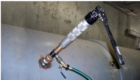
Model 7647 Corp-Stop Hot Tap Installation
