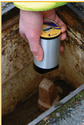
ADS Enigma Pod - Installation on Water Meter.
