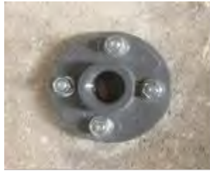
Securing Bracket to the Manhole Wall
