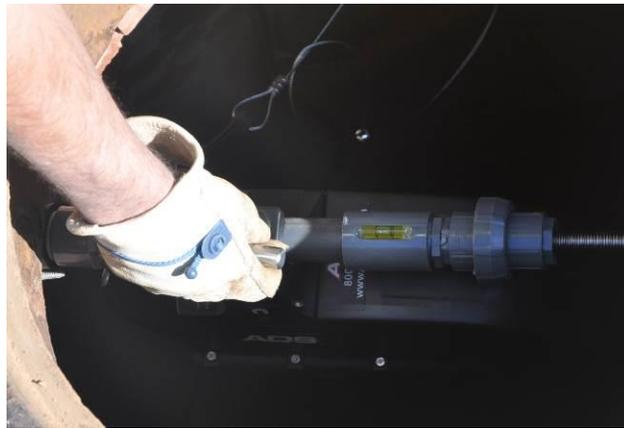
Placing Monitor on Mounting Bar
