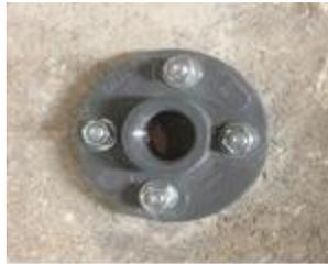
Securing Bracket to the Manhole Wall
