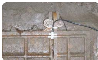
Zip tie in place
