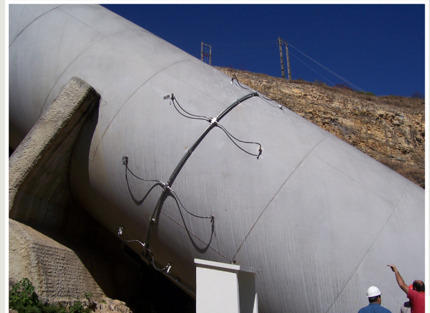
Feedthrough Installation on Penstock Pipe
