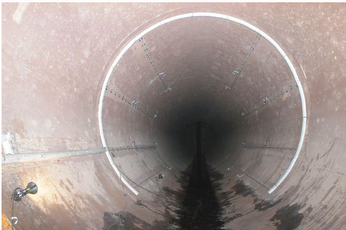
Internal Mount Installation on Penstock Pipe
