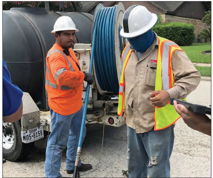
Photograph 1. Workers cleaning a collection system.
